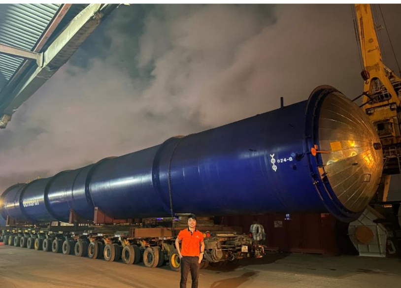
Handling Steam boiler: L38m x Dia 4,0m
