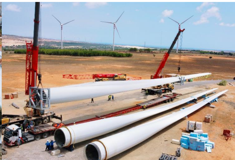
风力发电机叶片：L71m x W3.6m x H4.48m
